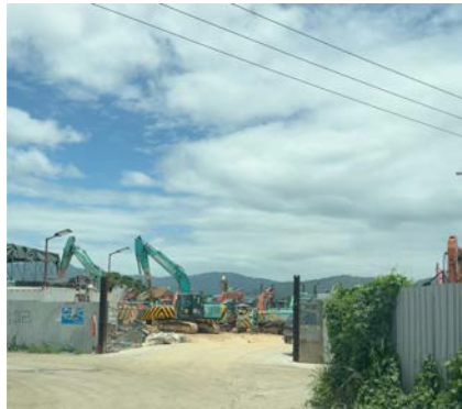
Figure: Brownfield operation next to A/YL-KTN/851. A large number of excavators are in operation, which may pose a danger to animals.
